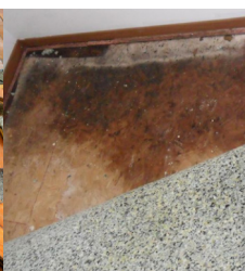
Leak Under The Floor
